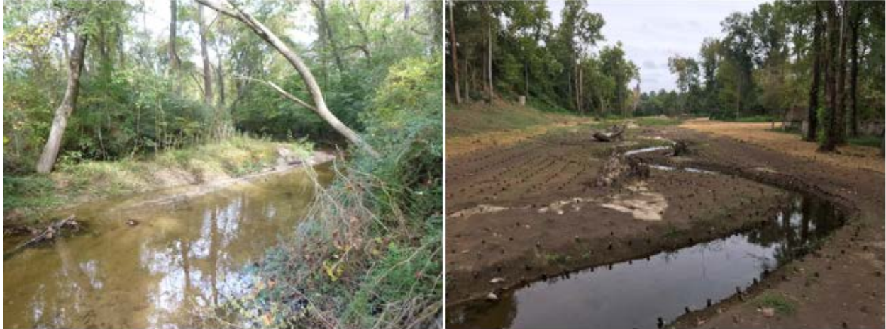
Image 2: Before (left, taken in 2017, provided by RES) and after (right, taken in 2019, provided by RES) stream restoration photos of Little Westham Creek restoration project (located on University of Richmond property). The relatively straight path of the creek was reengineered to flow in a meandering, S-curve in order to slow down the transport of nutrients and sediment. The slower flow rate also reduces the risk of flooding downstream.
