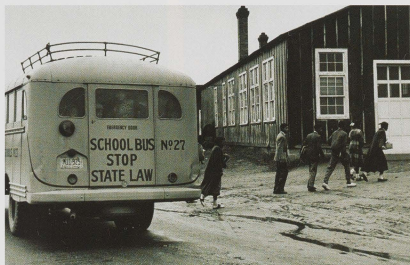
Students arrive for classes at a school building covered with tar paper.
