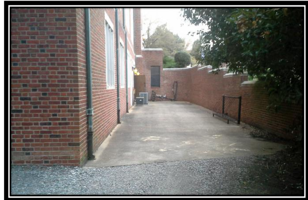
Figure 6.3 Cement floor where the rain barrels will be stored.
