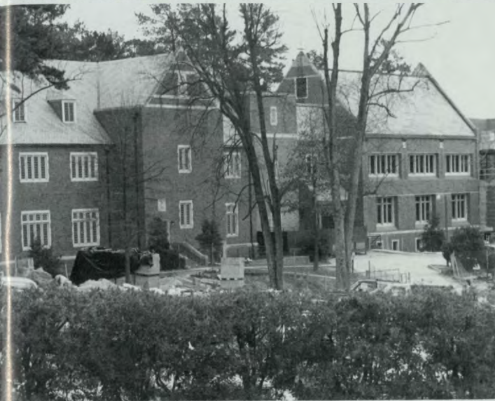
Construction on the Law School has everyone excited for upcoming endeavors.
