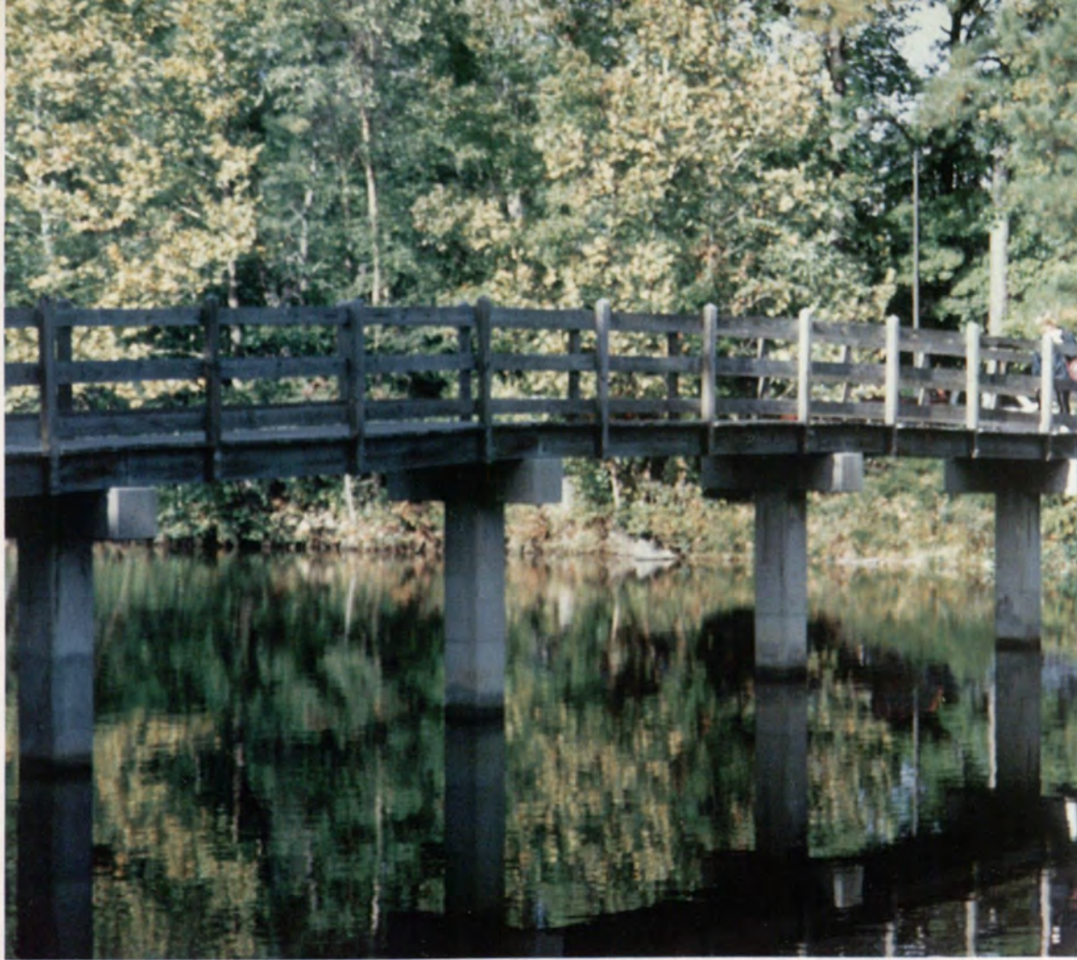
Spanning the lake, the bridge connecting the two sides of campus reflected the glistening lake. The bridge blended in well with the campus's forest atmosphere.
