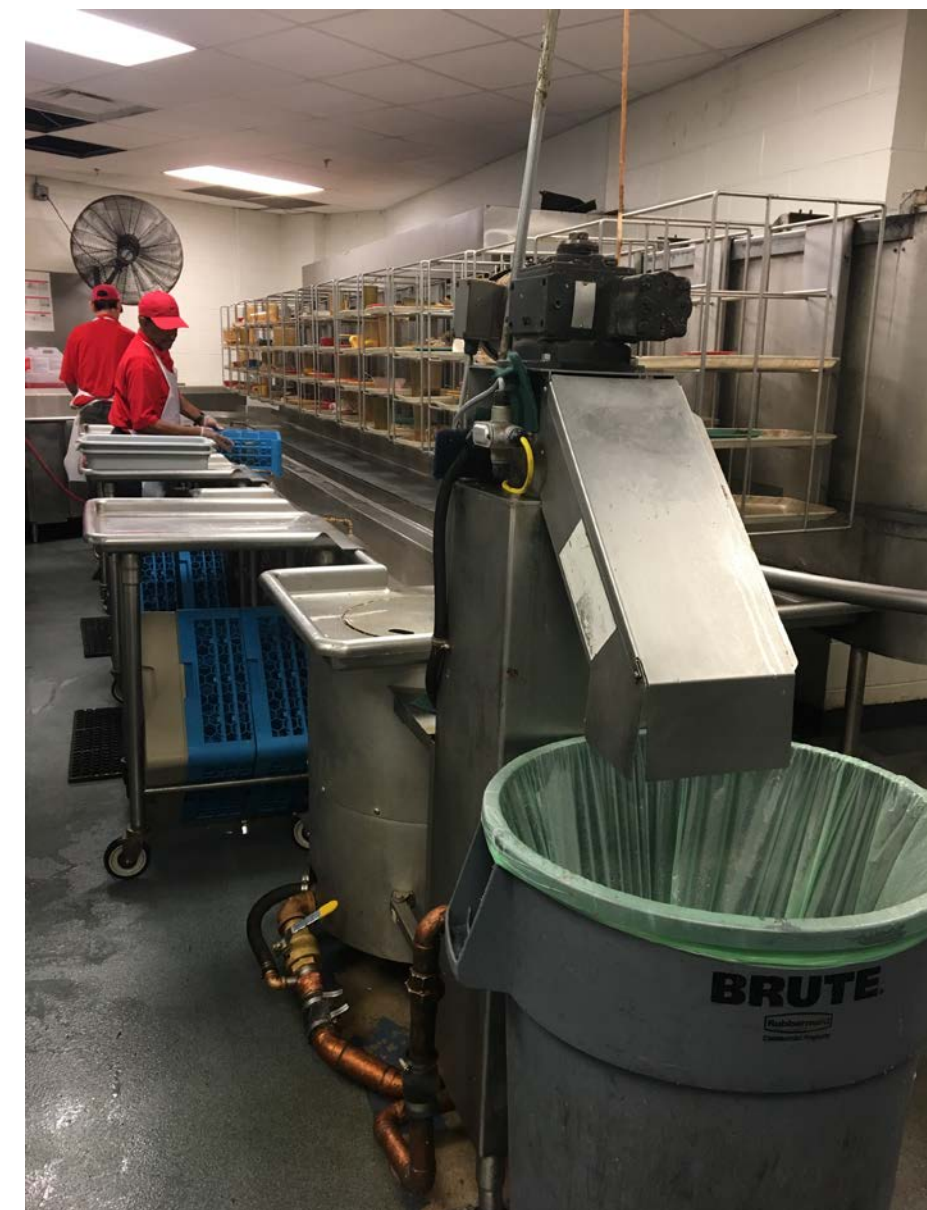
Figure 2: Dishroom at Heilman Dining Center and pulper that compacts waste (JP, 2017).
