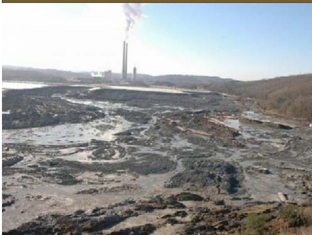
Aerial View of 2008 Coal Ash Spill, Kingston TN
