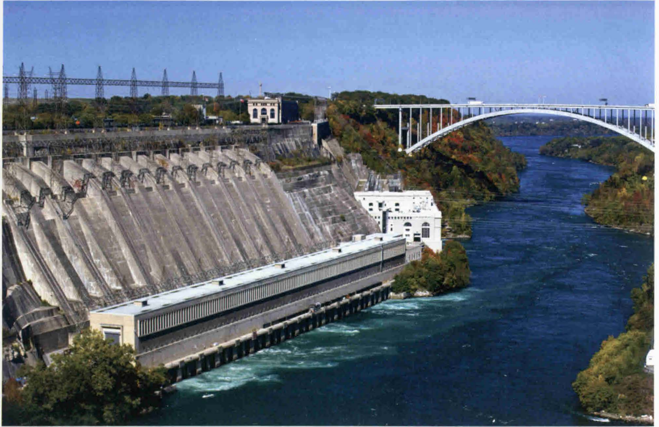
One of the Sir Adam Beck Hydroelectric Generating Stations, Niagara Falls, Ontario, with Lewiston-Queenston Bridge over Niagara River. (Performance Image/Alamy.) From Achieving Sustainability , 1E. © 2014 Gale, a part of Cengage Learning, Inc. Reproduced by permission. www.cengage.com/permissions .
